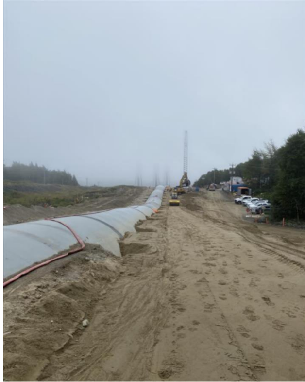
Figure 6: Placing Common Backfill on the South Side of Penstock
