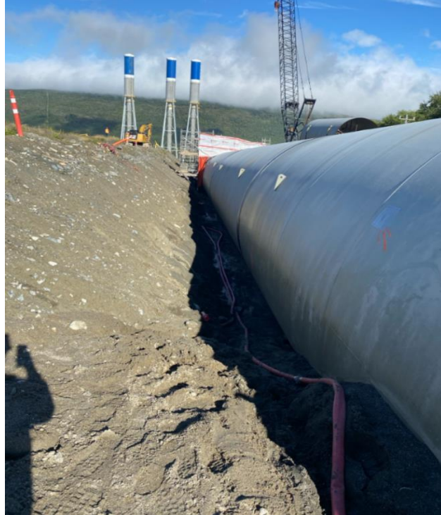
Figure 5: Placement of Bedding Sand to Springline Near Cans 18–21
