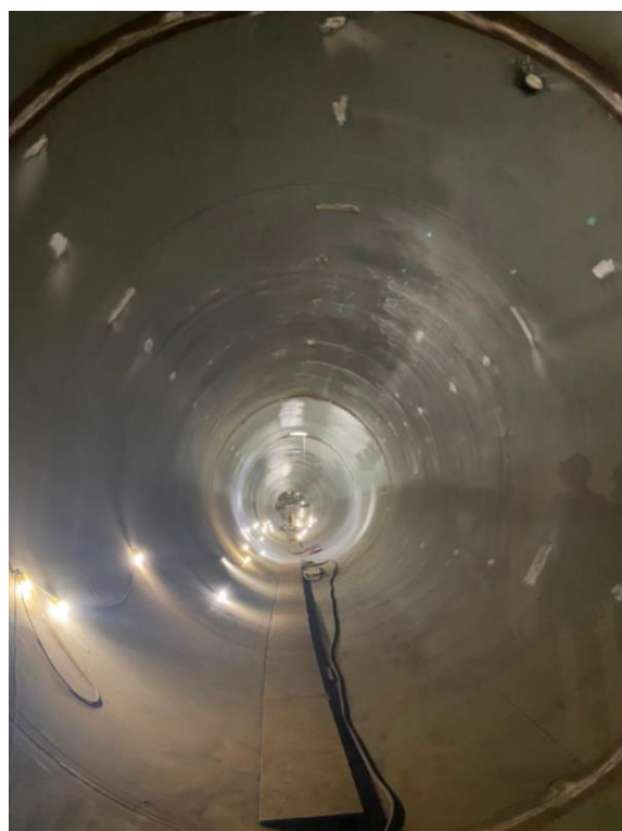
Figure 3: Internal Bracing Removed in New Cans
